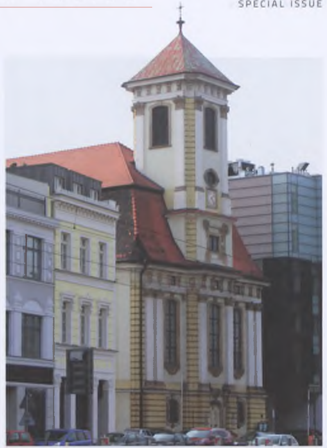
11. Evangelical-Augsburg Church of the Divine Providence, view from the northeast
