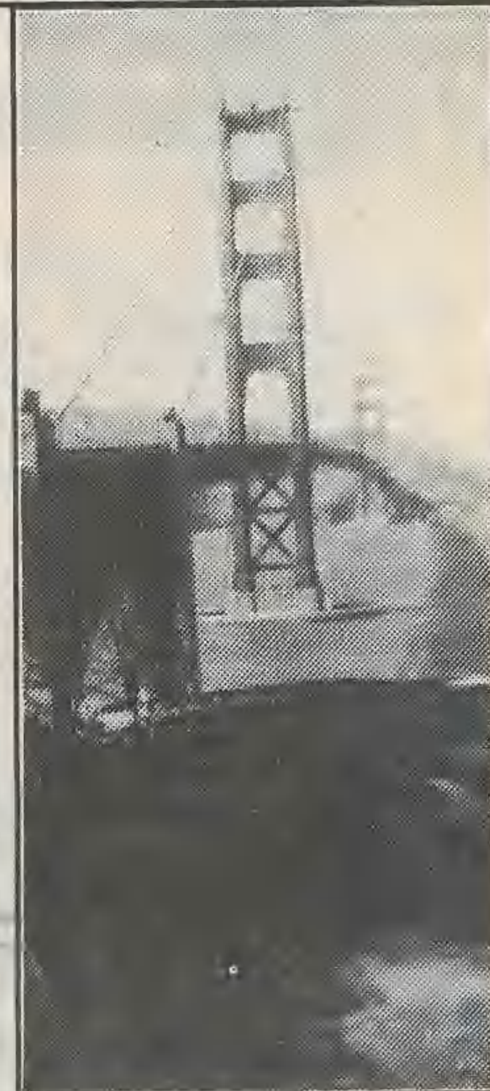
Golden Gate Bridge - San Francisco
